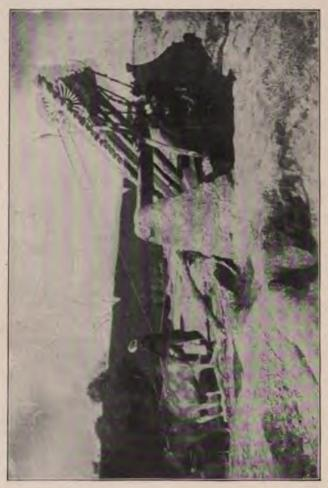
A modern water wheel (or cered) in Babylonia, illustrating ox-power machines of irrigation mentioned in the texts.
